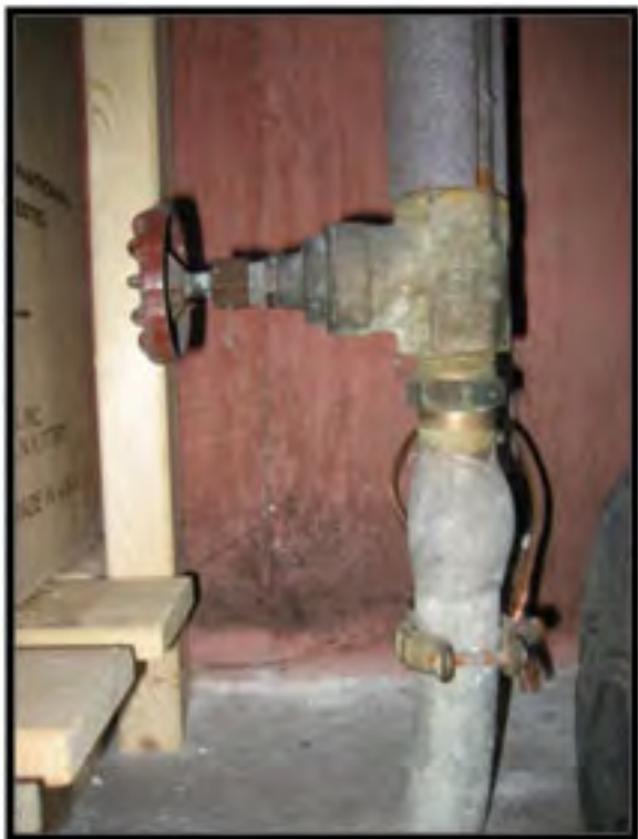
A Lead Service Line 39 Credit: EPA
